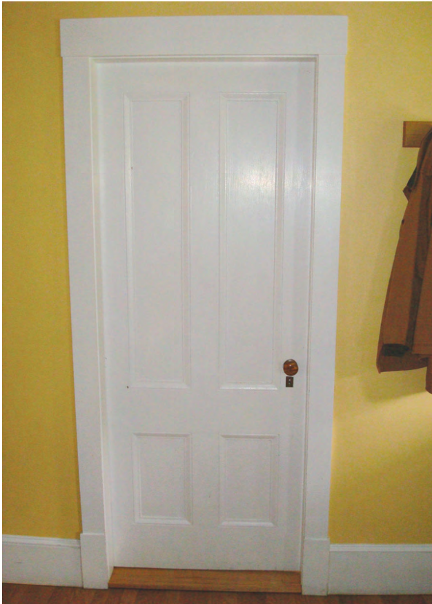
Photograph 3: Colonial Door —The most impressive “old guy” wood technology. Frames had virtually no cross-grains whereas panels which were cross-grained were allowed to slide into joints.
