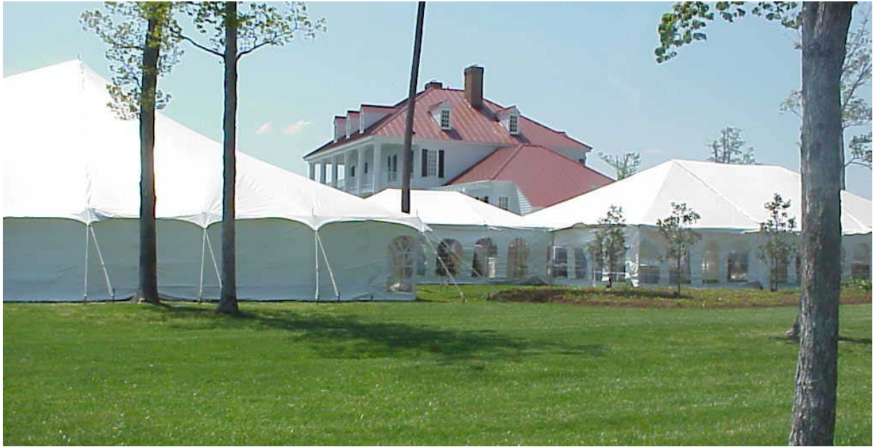
This photo fits the definition of a canopy, and at the same time, fits the building code definition of a tent:
