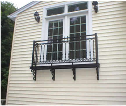
Landing size is 7 square feet service by a French door
