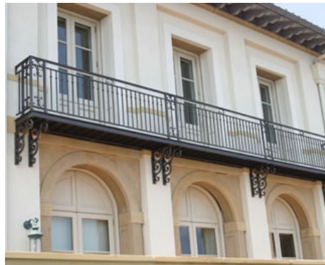
Landing size 57 square feet serviced by one French door in the center and two windows.
