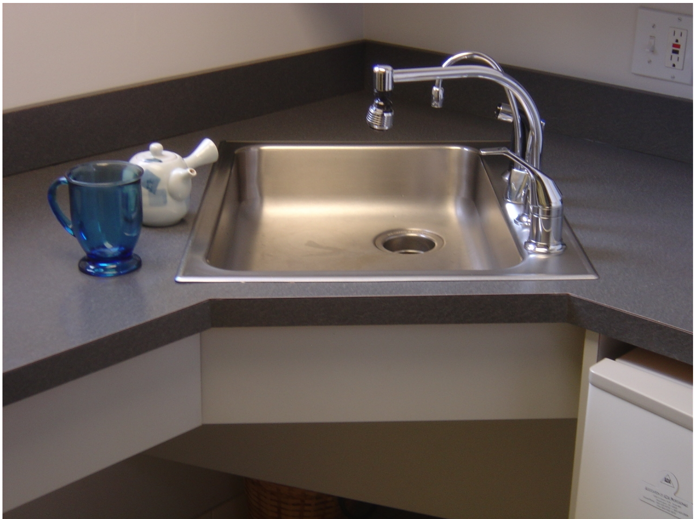
"Example of enhanced reach range faucets"
