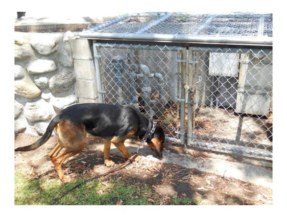
The photo taken above had a pressure vacuum breaker assembly installed on the supply side of a booster pump used for an irrigation system in a local park. The misapplication may also be a good indicator that the device has probably never been tested.
