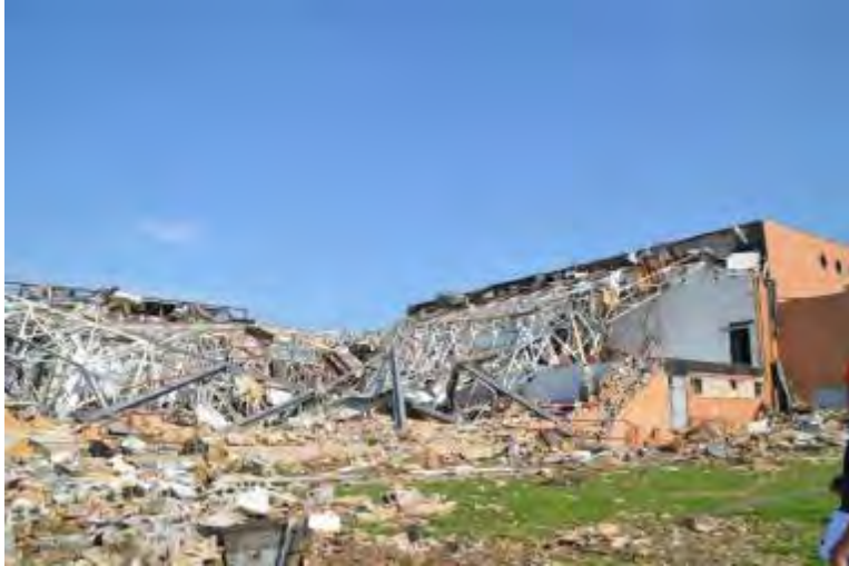
Figure 3 (Figure 6-56): View of the collapsed primary gymnasium of Joplin High School. The gymnasium collapsed through progressive failure.
