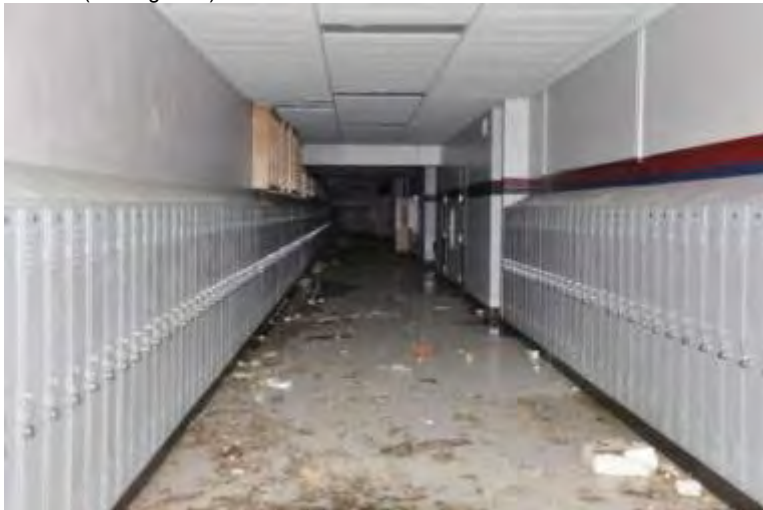
Figure 2 (Figure 6-52 of the MAT Report): View of a corridor designated as a tornado refuge area in Joplin High School. The debris was blown into the corridor during the tornado.
