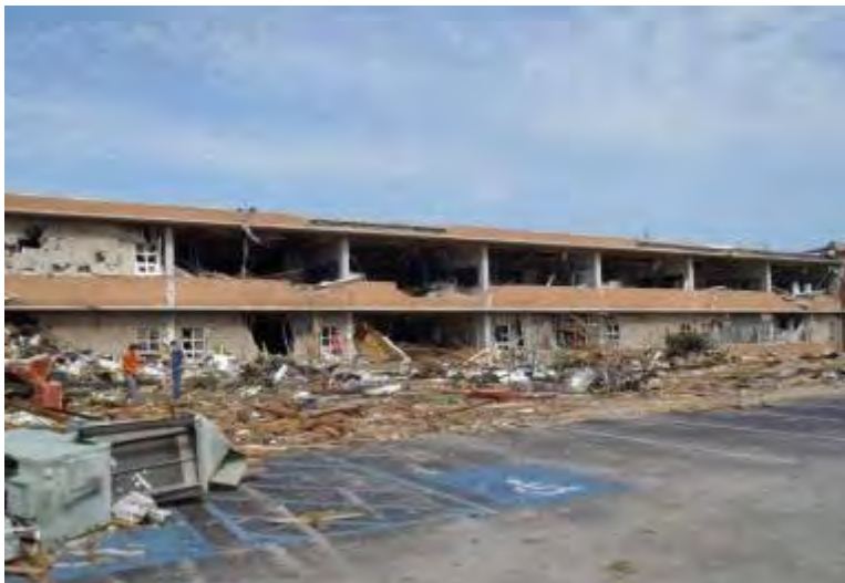
Figure 4 (Figure 6-53 of the MAT Report): North classroom wing damage of Joplin High School.
