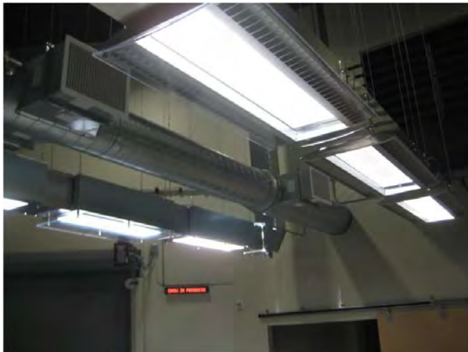
Sunlight being delivered to the interior space in an open ceiling (on the left) and in a dropped ceiling (on the right) by way of a sunlight duct system.
