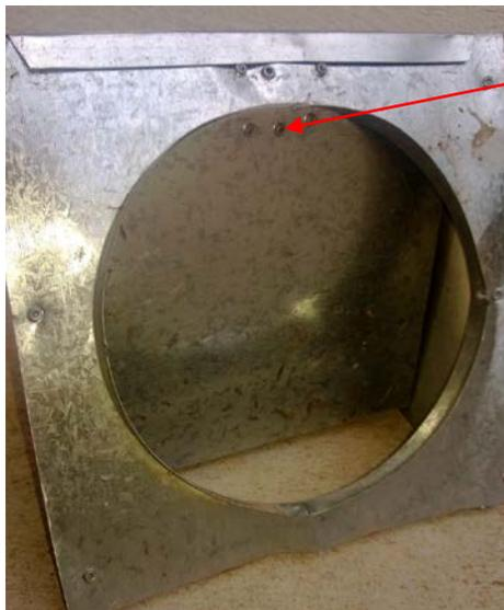
Images: Contractor-made gravity damper that came off a single family home built in 2000. Notice the canvas hinge (picture on right) attached with rivets (shown on left). It's clever, but I wouldn't count on it for life safety.
