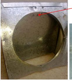
Images: Contractor-made gravity damper that came off a single family home built in 2000. Notice the canvas hinge (picture on right) attached with rivets (shown on left). It's clever, but I wouldn't count on it for life safety.
