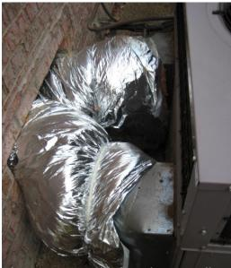
The opening in the foundation wall is not wide enough for the HVAC unit.
