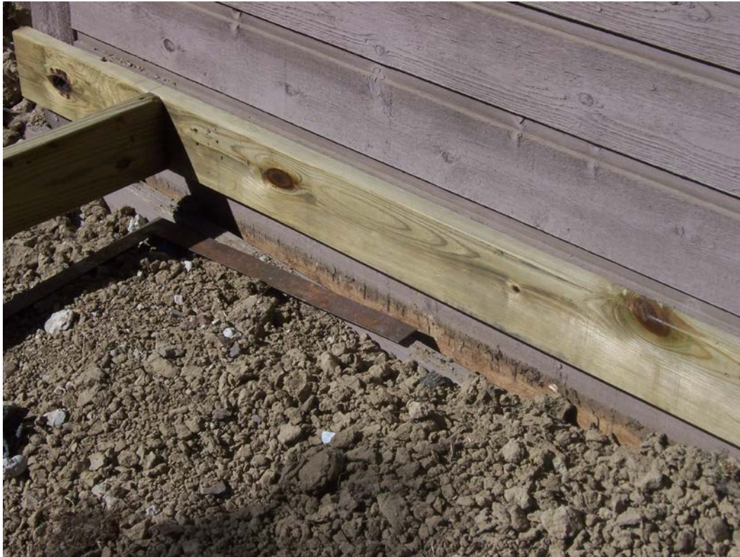
The contractor attached it over siding with no flashing, and buried the siding with about eight inches of dirt excavated from the piers.
