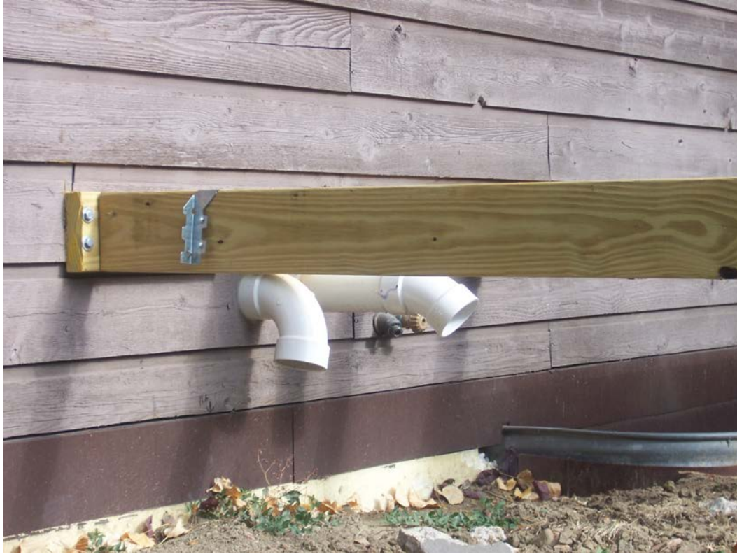
The contractor attached it over siding with no flashing, and buried the siding with about eight inches of dirt excavated from the piers.
