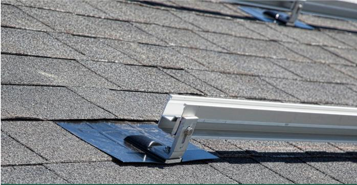
Figure 6. Flashing and sealing
