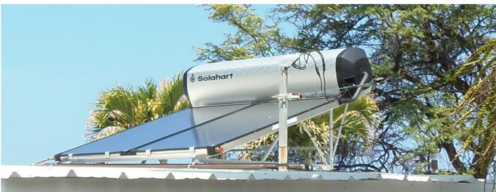
Figure 4. Roof-mounted thermosiphon solar water heating system
