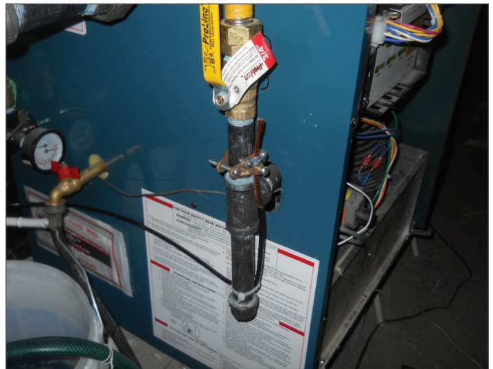
Example of Bonding at the Drip Leg
