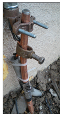
Grounding Electrode Connection
