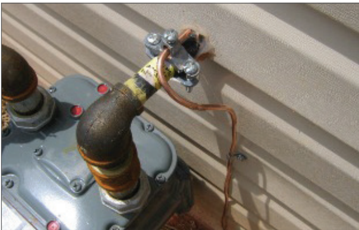
Example of Bonding at the Service Entrance
