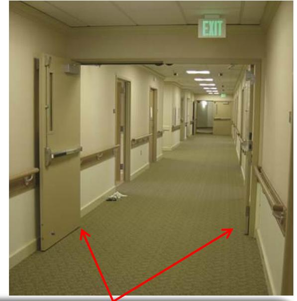
Cross corridor doors as part of smoke barrier held in place with magnetic hold-open device released by smoke detectors or fire alarm
