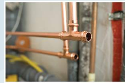
Press-connect copper fitting
