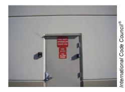
Fire sprinkler riser room is identified and a lock box is provided to allow fire department access.
