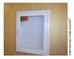
This hose cabinet previously contained hose and nozzle for occupant use. These items have been removed and the remaining connection is compatible with the fire department hose fittings.
