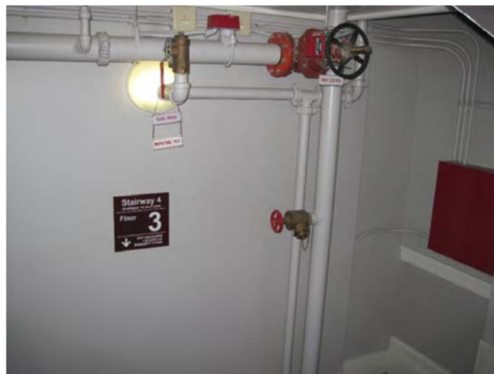
FIGURE 9-9 Standpipe system.
