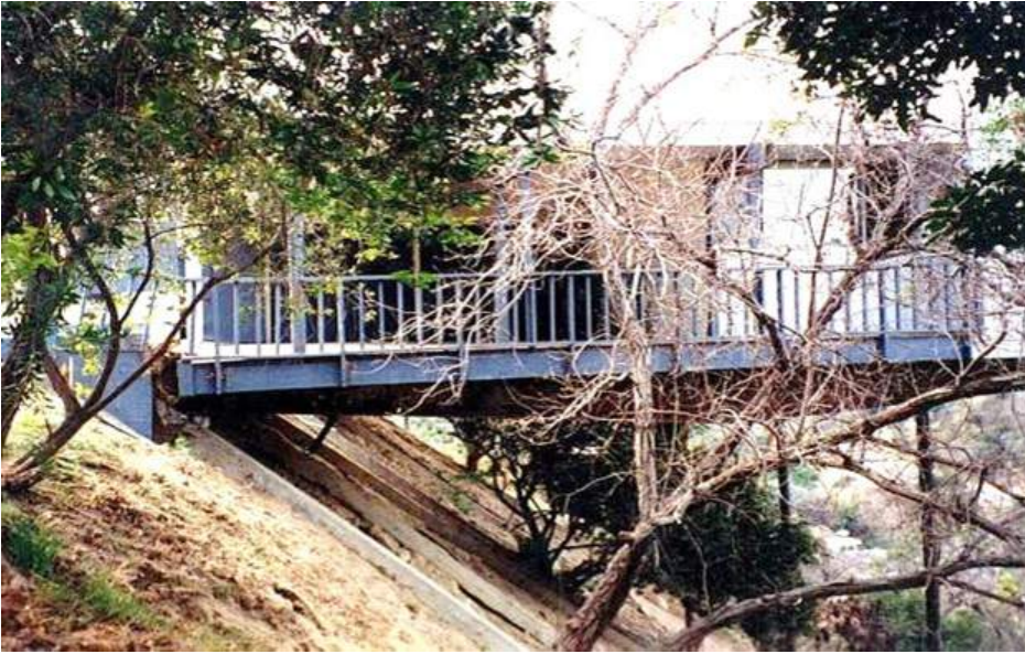
Figure 3. Hillside dwelling pulled away from uphill foundation in the 1994 Northridge, California Earthquake (Credit: City of Los Angeles Department of Building and Safety). Red arrow shows location where floor framing has pulled six to eight inches away from the uphill foundation.
