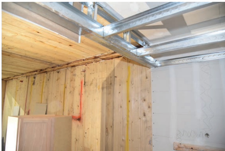
Concealed spaces must be protected.
