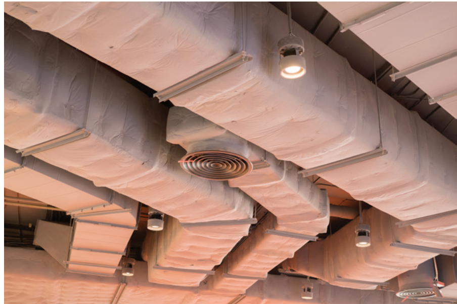
Duct insulation
