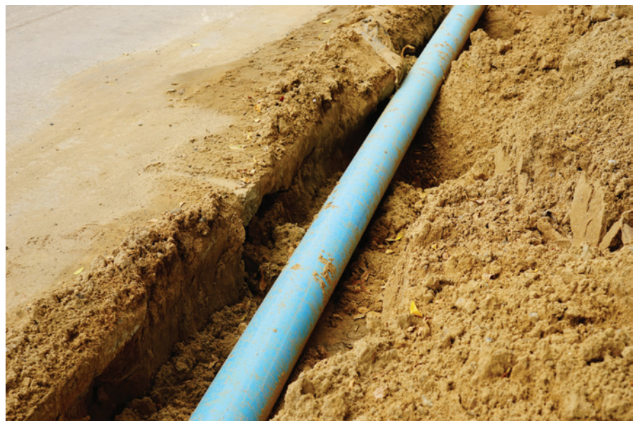
Tracer required for underground nonmetallic water service pipe
