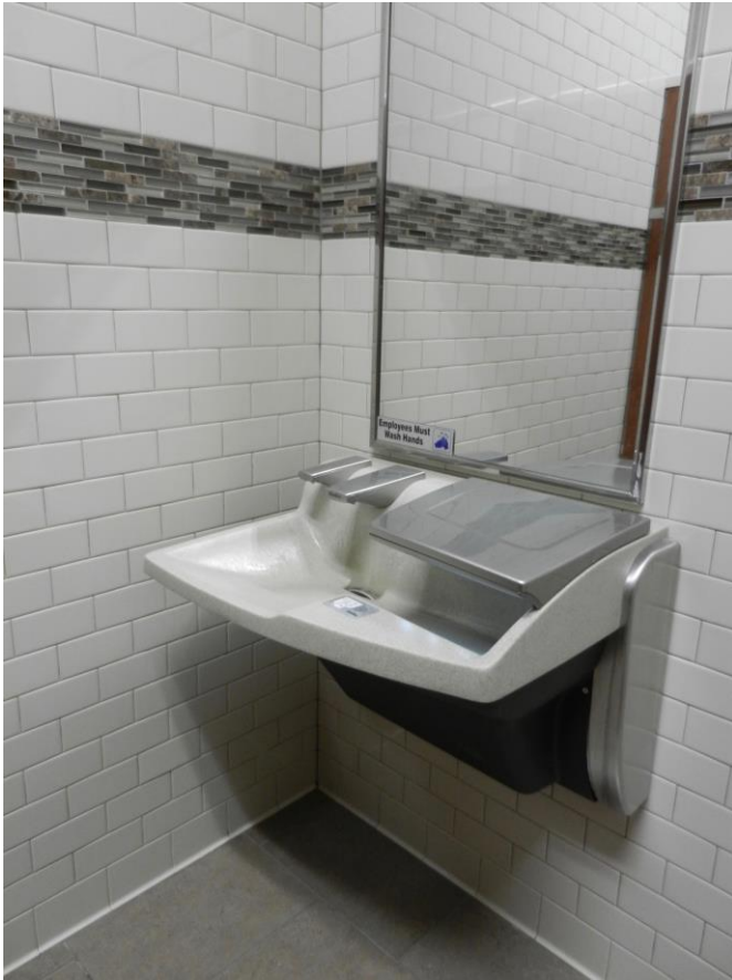
Hand dryer in the lavatory.
