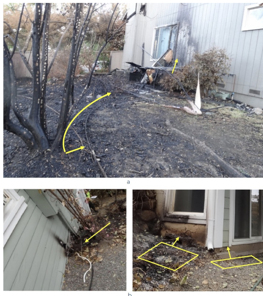
Figure 1. Example of vegetation in small amounts located in Zone 0 creating a pathway for fire spread: (a) Wood mulch provided a pathway for fire to get close to the building and ignite a hot tub during the Glass Fire (2020) in Napa and Sonoma Counties, California; (b) Ground-level plants during the Glass Fire (2020).
