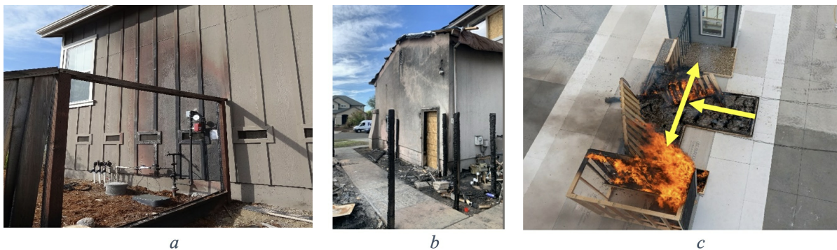
Figure 1. Examples of combustible fencing providing a pathway for fire to the house, damaging the noncombustible siding.
