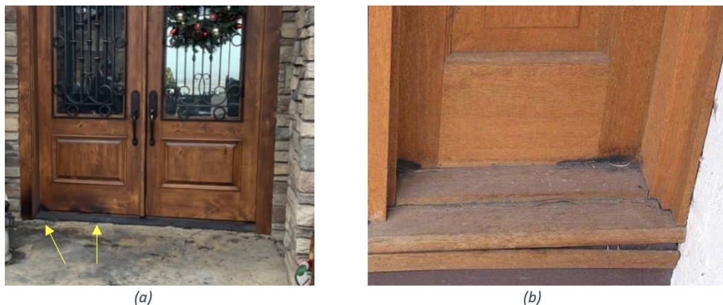
Figure 1. ignition from accumulation of embers and debris at the base of the door.
