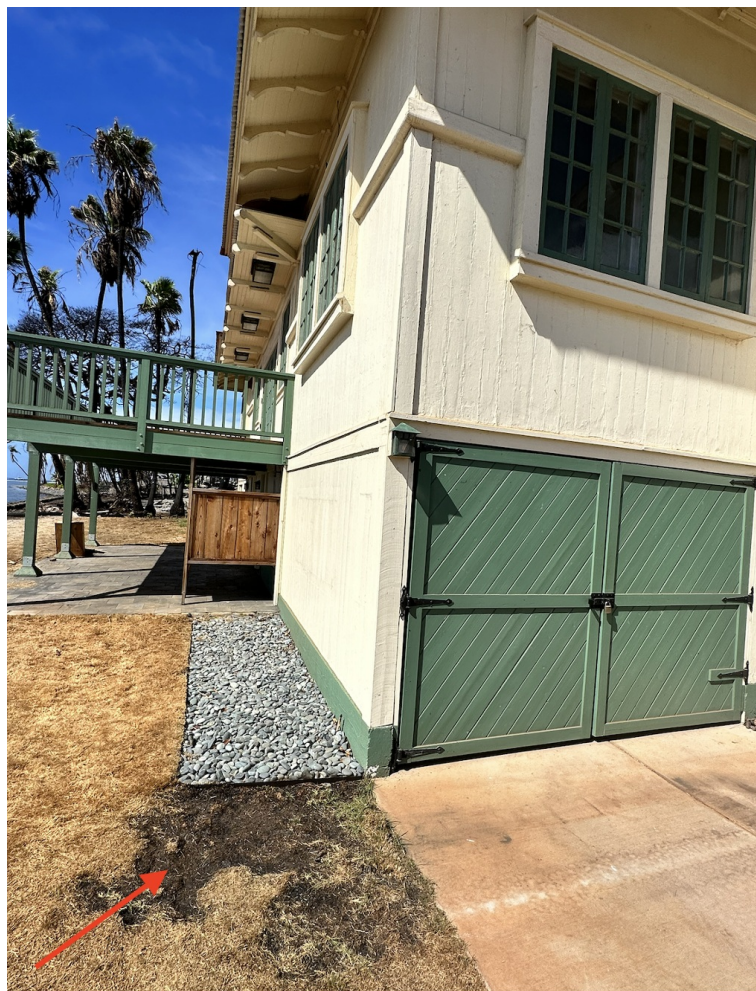
Figure 2. Noncombustible mulch breaks the fuel path in Lahaina wildfire. Photo courtesy Milad Shabanian, IBHS.
