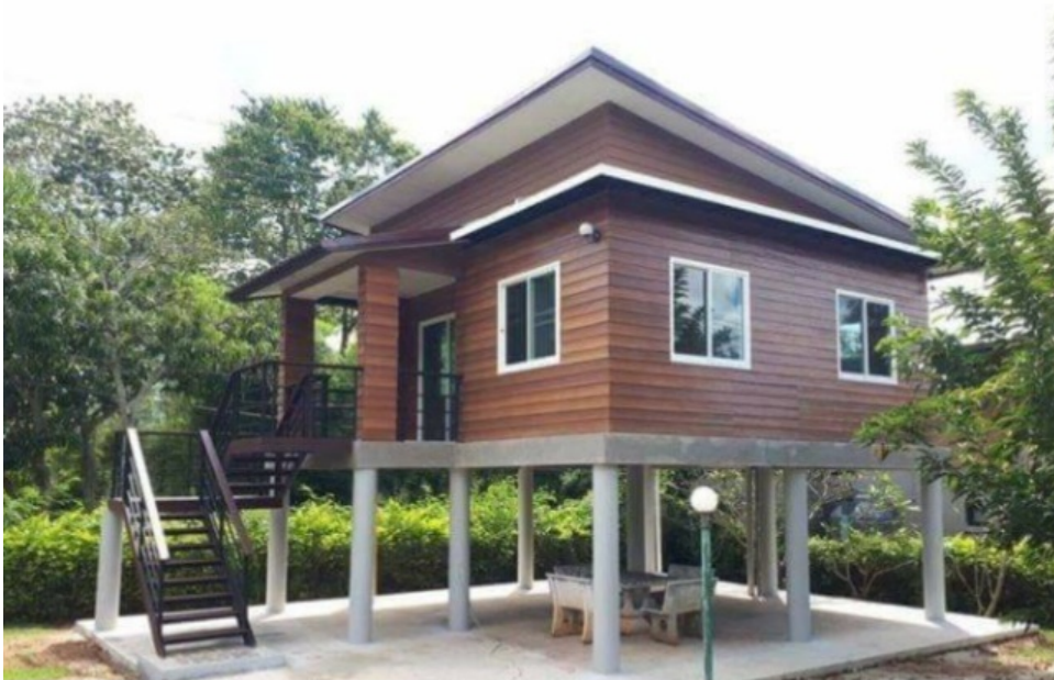
Figure 1. Usable unenclosed underfloor areas.
