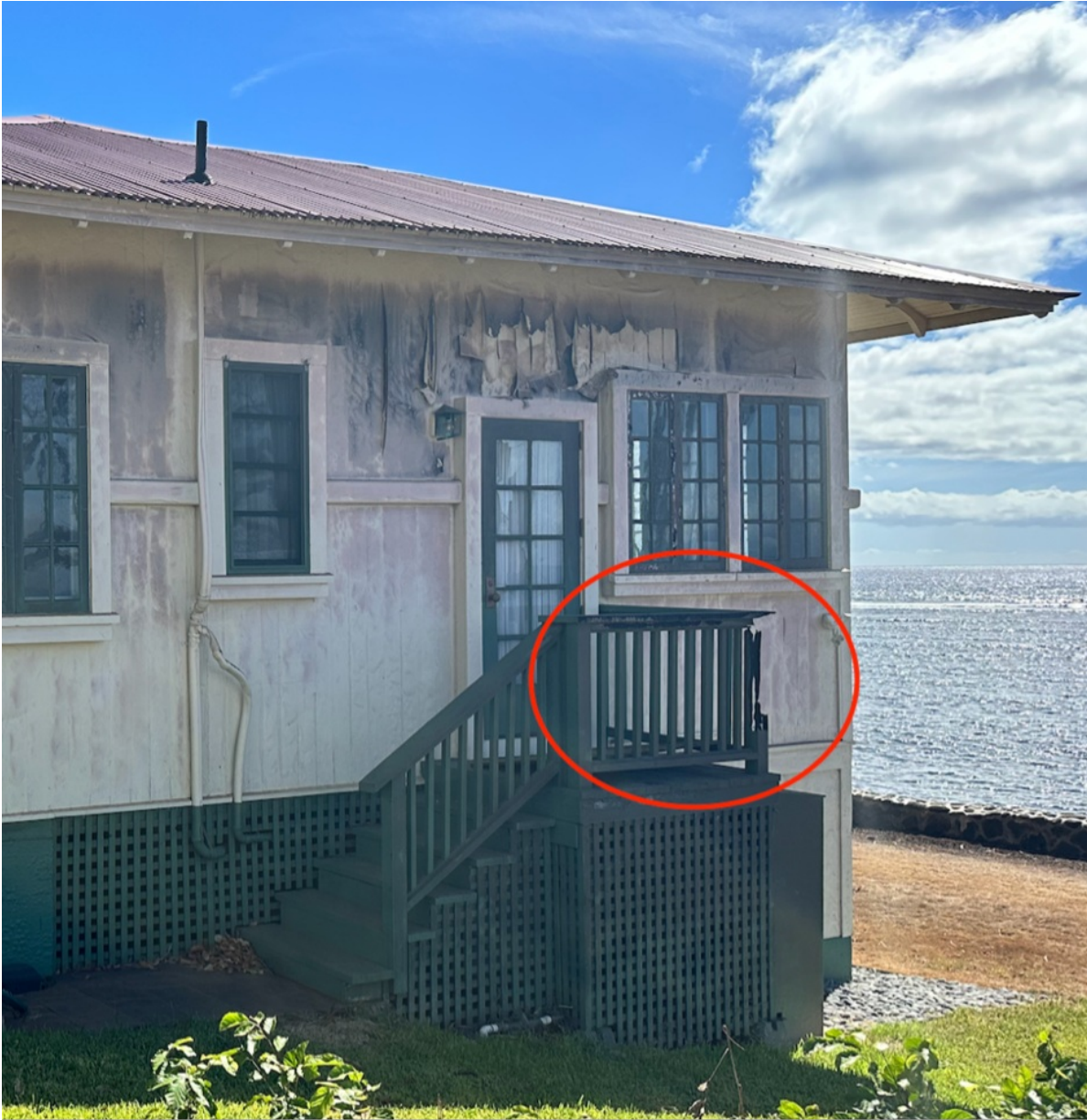
Figure 1. Nonconforming attached accessory structure (stair). Photo by Milad Shabanian, IBHS.
