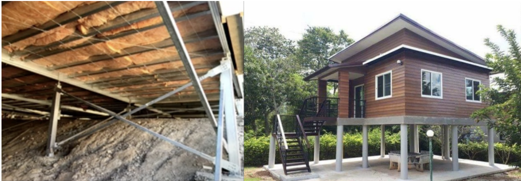
Figure 1. Noncombustible unenclosed underfloor areas.
