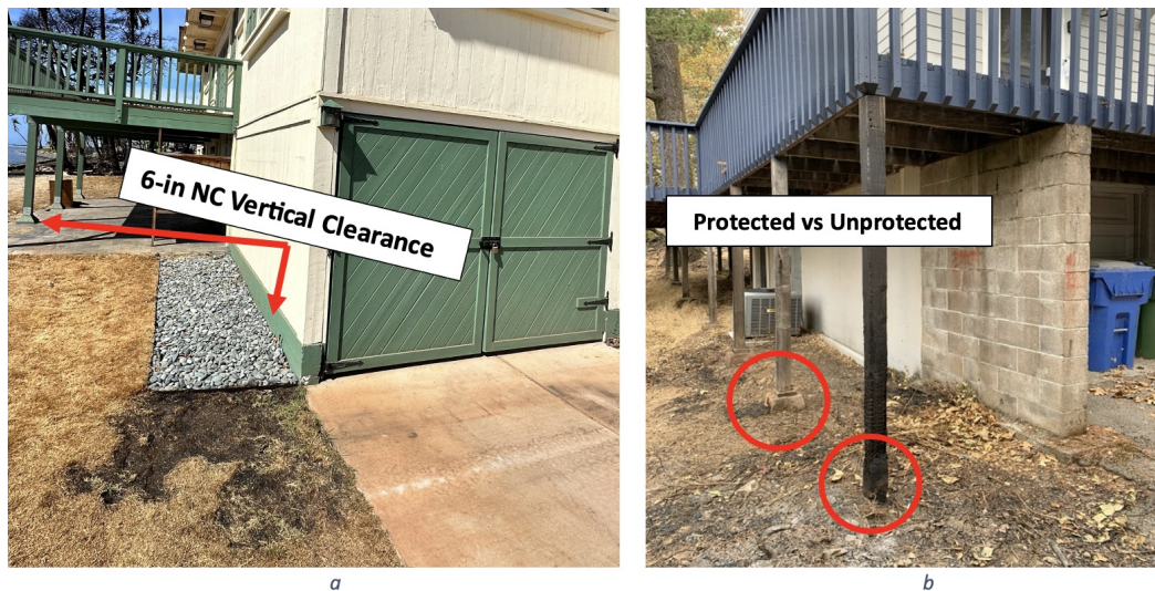
Figure 2. 6-in Noncombustible vertical clearance at the base of exterior walls and underfloor area columns: a. Lahaina Fire 2023 (Photo courtesy Milad Shabanian, IBHS), b. Glass Fire 2020 (Photo courtesy Steve Hawks, IBHS).
