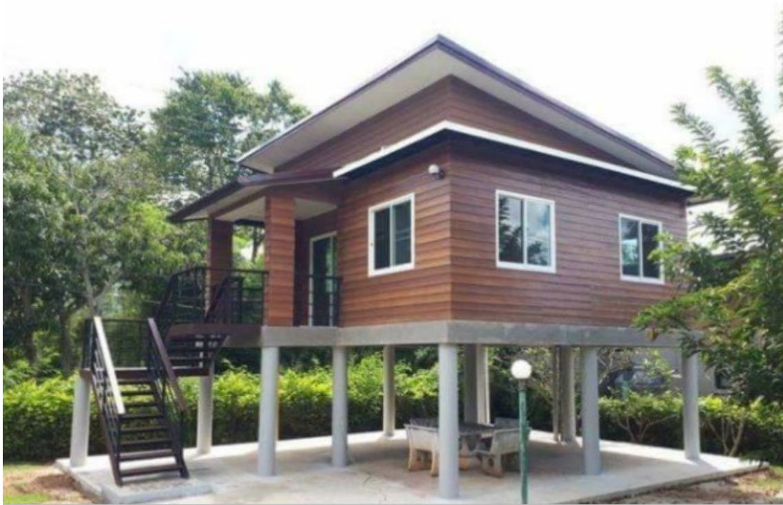
Figure 1. Usable unenclosed underfloor areas.
