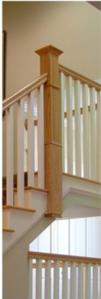
Handrail to Post as permitted by code
