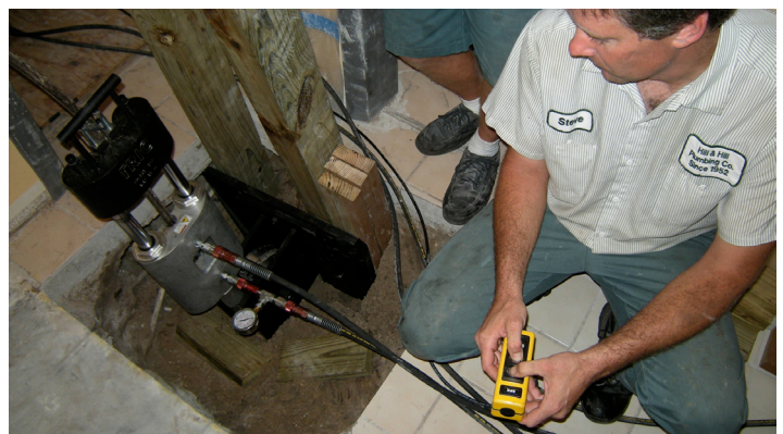
Trenchless equipment puller set up in the pulling pit
