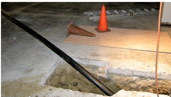
New HDPE pipe attached to bursting head enters existing pipe
