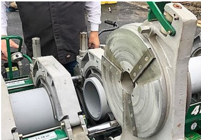
The fusion joining process of HDPE pipe prevents future root intrusion Photo from Trenchless Equipment
