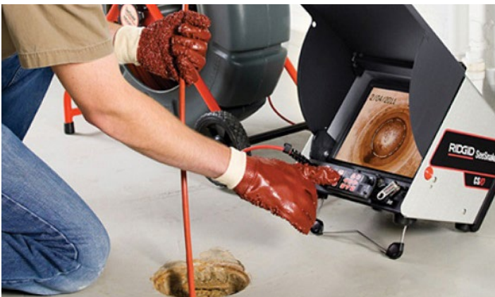
Drain Camera in Use
