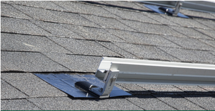
Figure 6. Flashing and sealing
