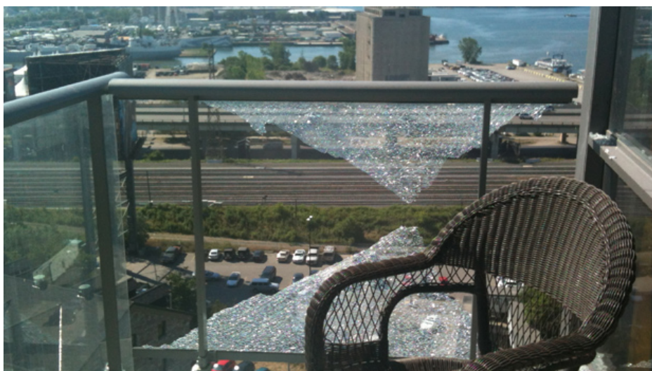
July 2012 - Broken tempered glass assembly 15th floor condo at 33 Mill Street, in Toronto.
