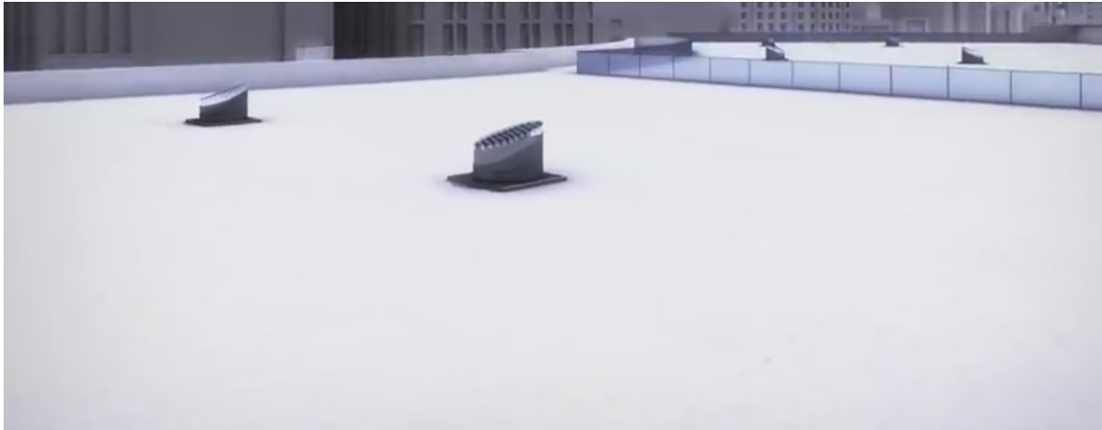
Roof top solar collecting devices used in a sunlight delivery system.
