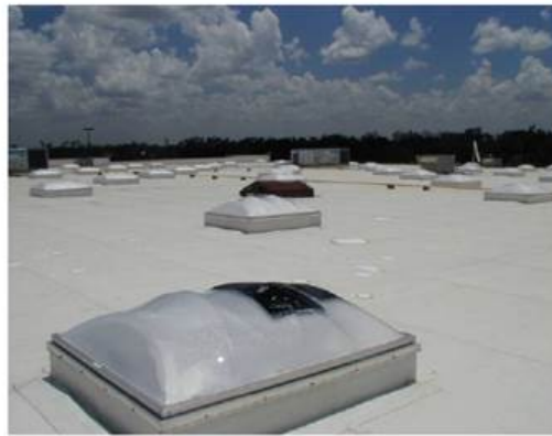
3-09-3. Large retail building. Broken skylights became wind-borne debris, puncturing roof membrane—SE view.
