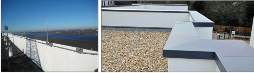
Examples of coped parapets as required by 1503.3.1.
