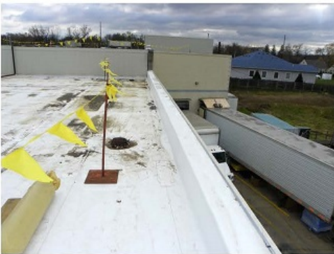
Hyvee Iowa Fascia on 18" parapet condition
