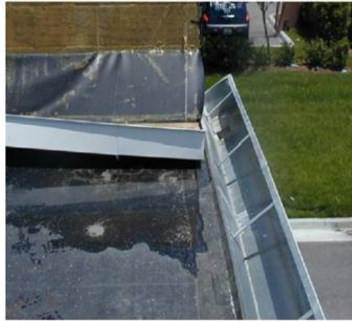
3-08-2. Small retail building. Roof view of lifted gutter and metal edge. Note roof membrane has not peeled back.
