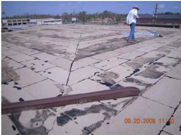
2.11-2. Membrane peeled away from the insulation and detached from the roof in most
