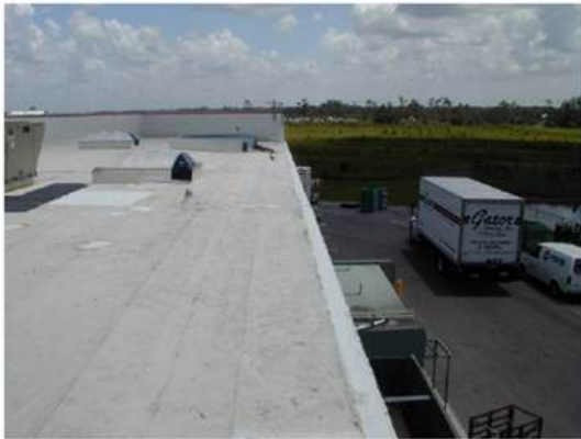
3-09-2. Large retail building. Gutter metal blew across the roof, puncturing the roof membrane and breaking skylights.
