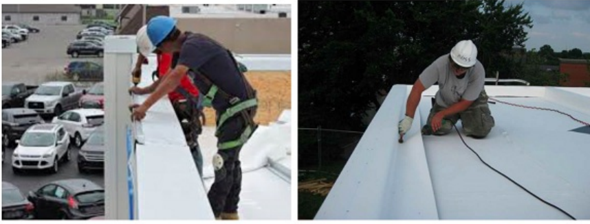
Examples of coped parapets as required by 1503.3.1.
