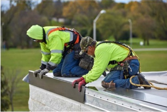
Fascia on 6" wide by 4" high "Parapet"
