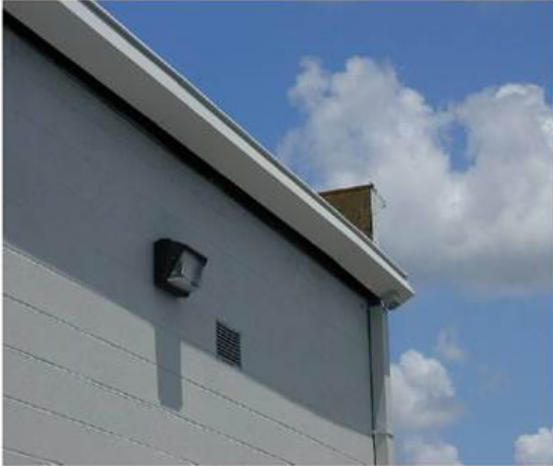
3-08-1. Small retail building. Close up of windblown, deflected gutter.
