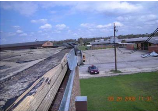
2.11-10. Photo of gutter/cleat attachment is a good example of damage progression.
