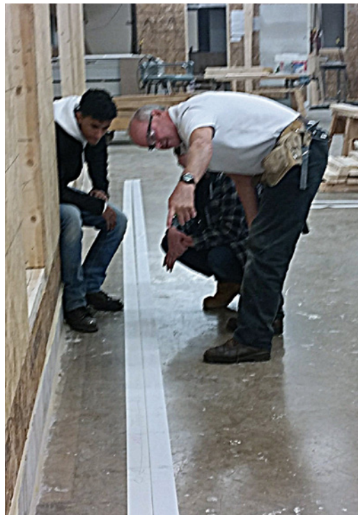
Harry Hintz showing students how to lay out wall plates.
