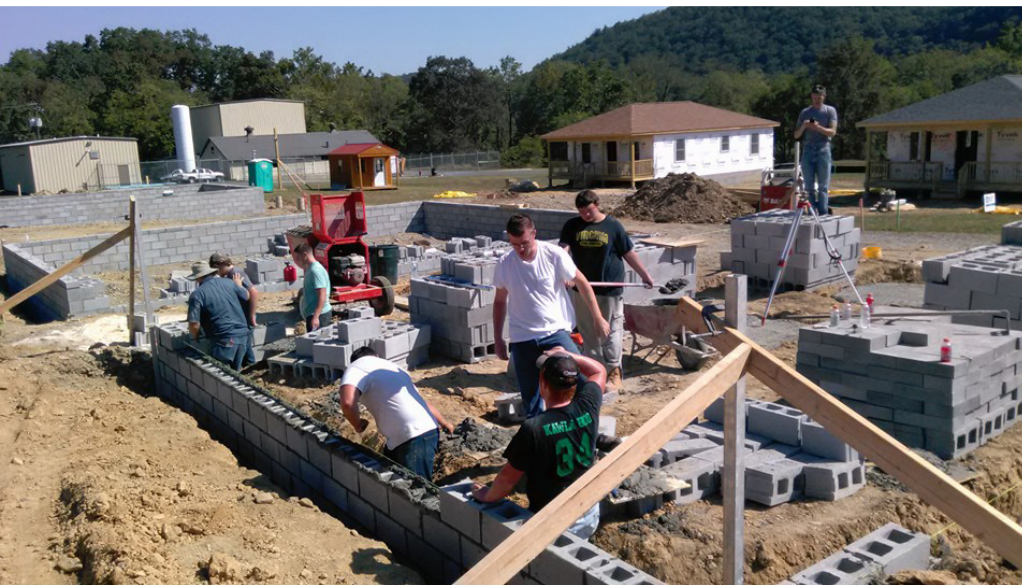
Top image: Tazewell mason instructor Robert Steele shows students how to square up foundation on footing and set story poles. Bottom image: With work assignments in hand, students get to work.
