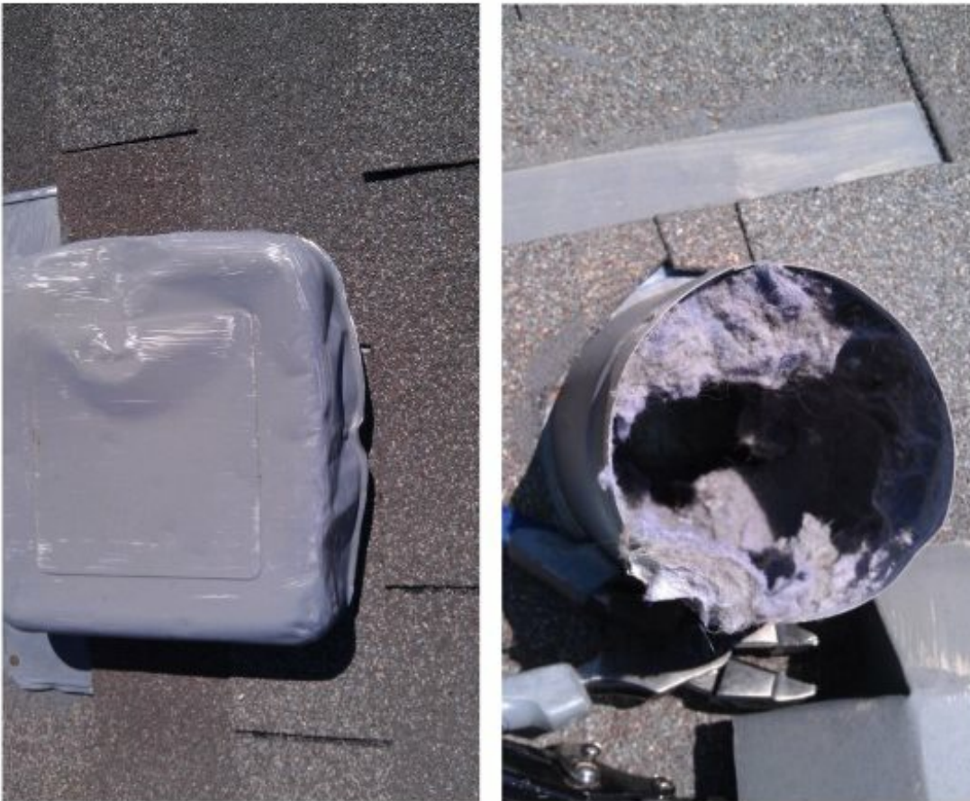
Examples of vent caps that duct cleaners wrongly disassemble to gain access.
