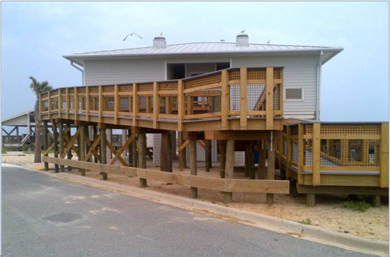
Figure 3. Florida, Gulf Coast, flood Zone V. Ramp built after original elevator determined to be unsustainable due to significant maintenance problems.
