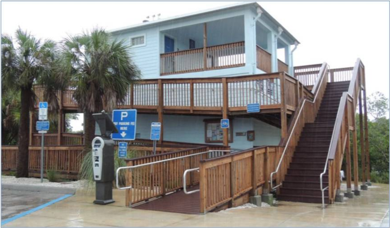
Figure 1. Florida, flood Zone V. Ramp wraps around entire building. Has composting toilets, battery and solar electric system, emergency plan requires pumping out tank and filling with clean water.
