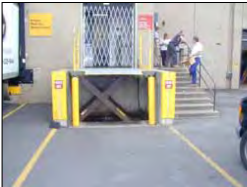
• Scissors lift in 3-sided pit at loading dock # 1
