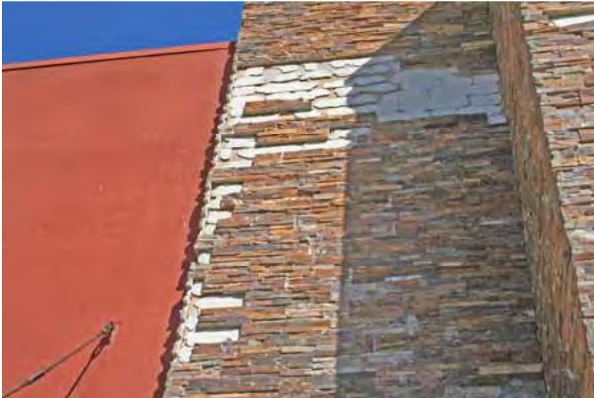
Here, only a few units have fallen, so far. No mechanical attachment.
