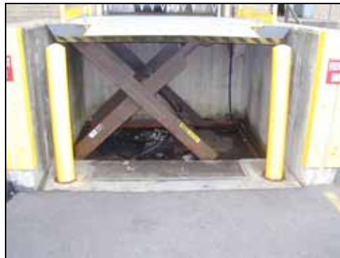
• Scissors lift in 3-sided pit at loading dock # 2
