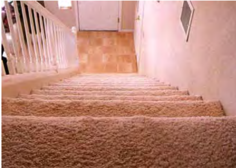
Figure 2. Typical Dwelling Unit Stairway with the Systemic, Top-of-Flight Defect.
