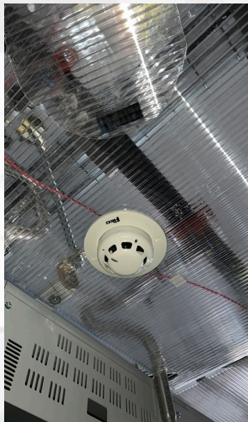
Figure 4-4 There will likely be several smoke detectors, like this one, mounted at ceiling level in larger enclosures.
