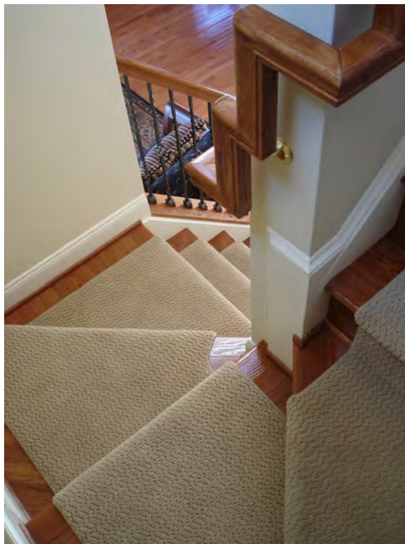
Figure 1. Crude fittings permitted at winders by relaxed Code rules.
