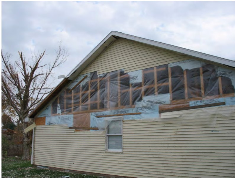
Figure 1. – Foam and vinyl wall covering failure. (Storm damage – Southern IN, 2005)
