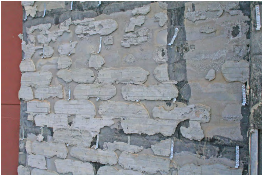
Another project: Upon stripping the façade, it appears an attempt was made to “anchor” the units, but it was clearly unsuccessful
