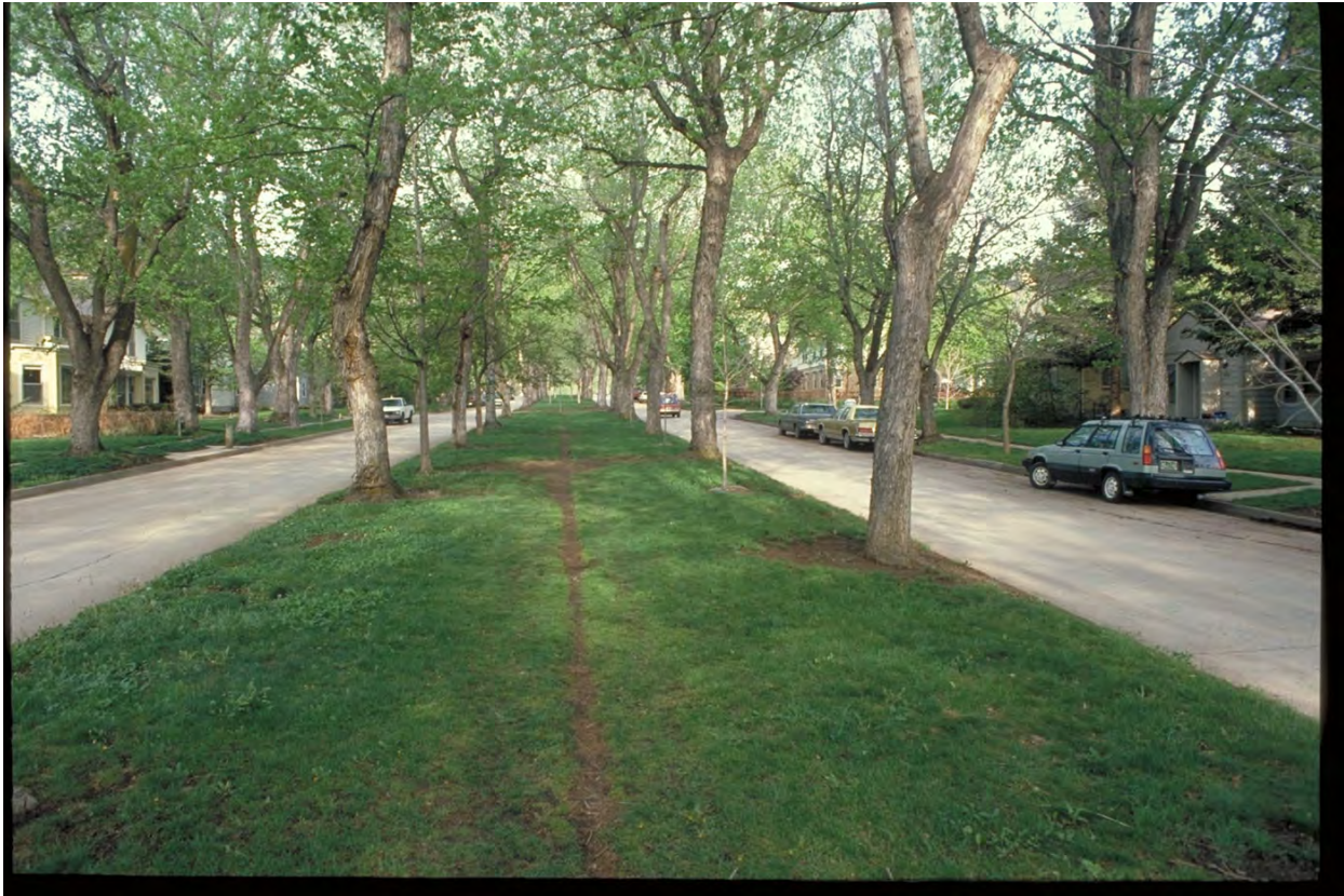
An example of a roadway with a raised median and approximately 17 feet of clear width on each side of the median. Photo: median.jpg
