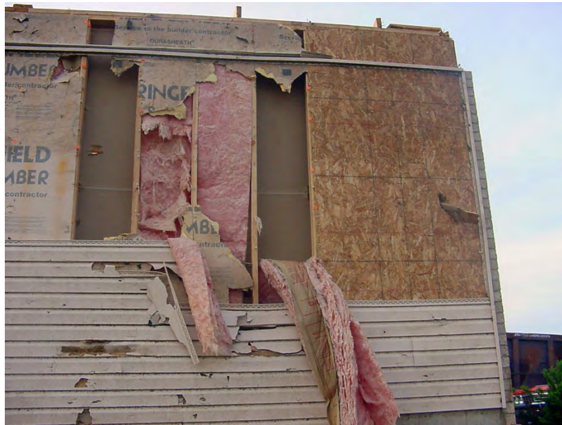
Figure 2 – Foam and vinyl wall covering failure while wall bracing panel remains. (Storm damage, Springfield, MO, 2006)
