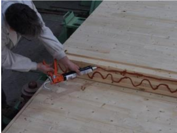
(a) sealant along spline joint
