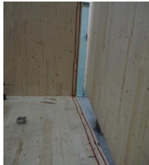
(e) sealant along butt joint
