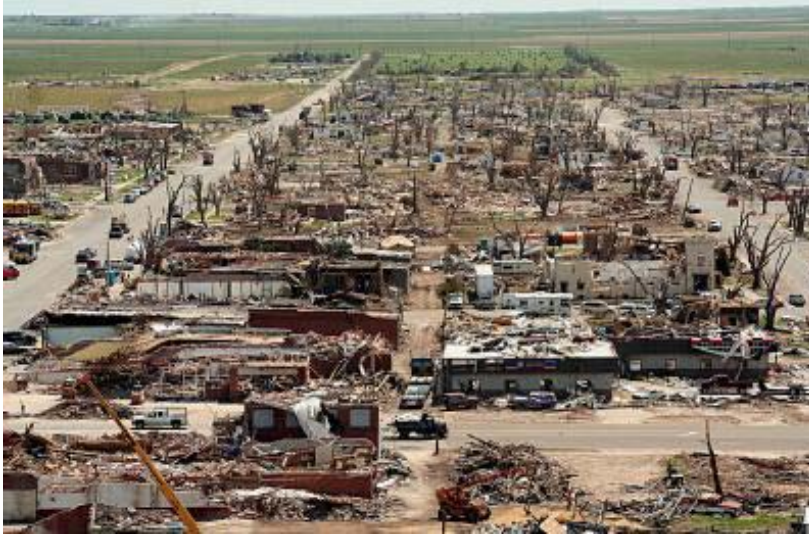
Tornado damage – FEMA
