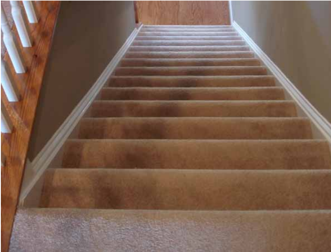
Figure 3. Dwelling Unit Stair Very Likely Not Having the Systemic, Top-of-Flight Defect.
