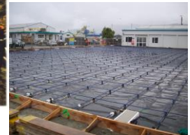
Size, depth, reinforcing, pads, holdowns
