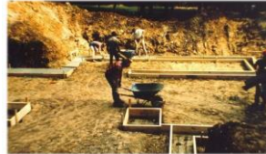
Size, depth, reinforcing, pads, holdowns
