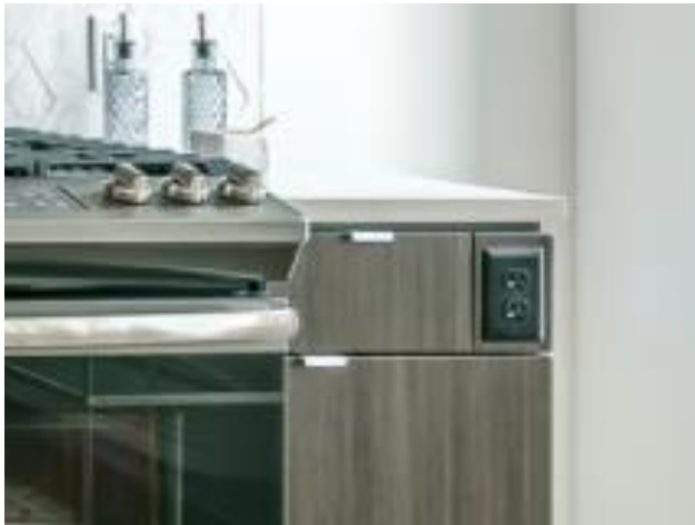
Outlet in front of cabinet where drawer width is reduced.
