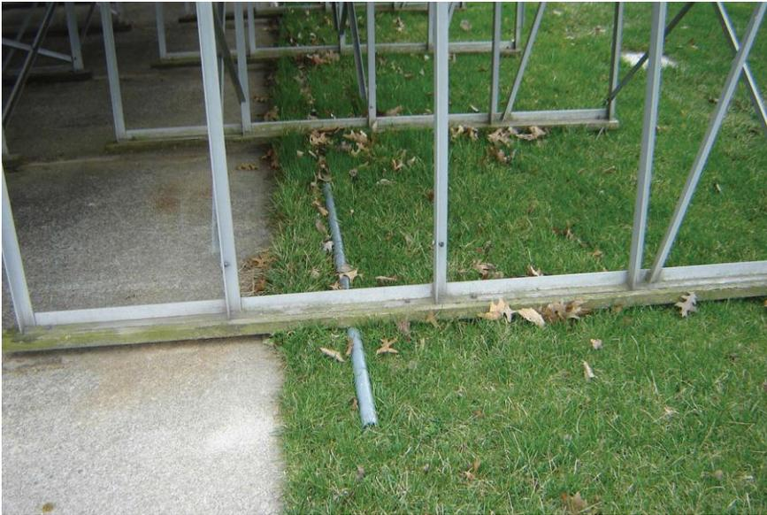
Mudsill stand blown off concrete slab foundation
