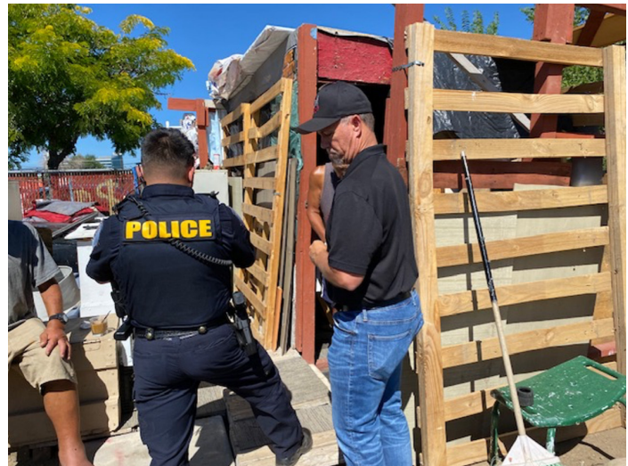
Inspecting Illegal Shed
