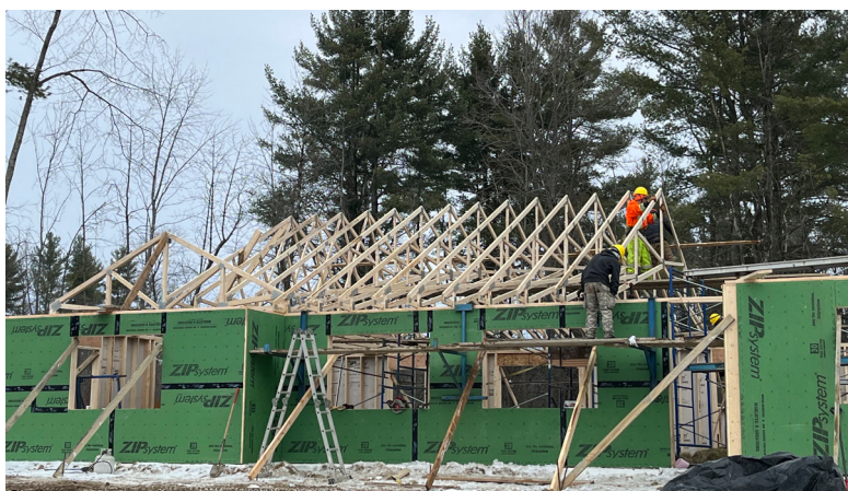
Trusses – courtesy of St Regis Mohawk Tribe (THPO)
