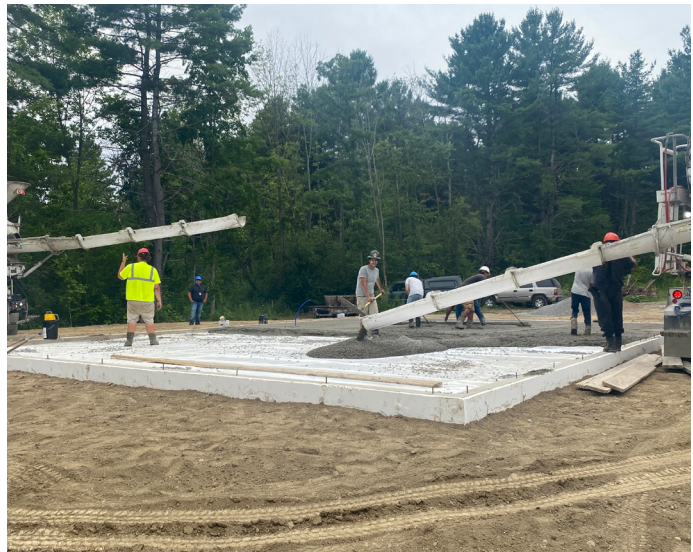
Concrete pour – courtesy of St Regis Mohawk Tribe (THPO)
