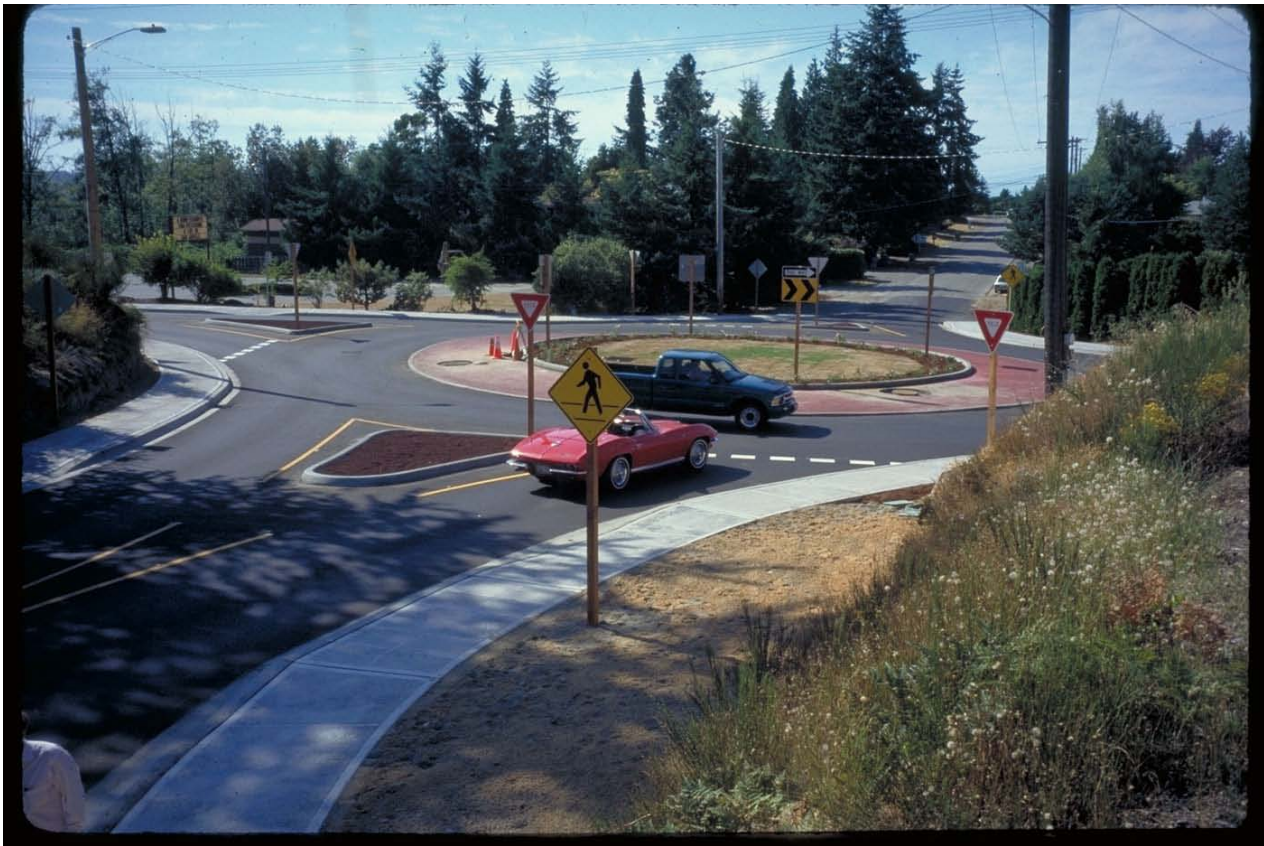
A typical modern roundabout in University Place, WA. At the roundabout entry, the clear width provided is only approximately 13 feet: this is an intentional design element to keep vehicle speeds low. Photo: IMG0032.jpg
