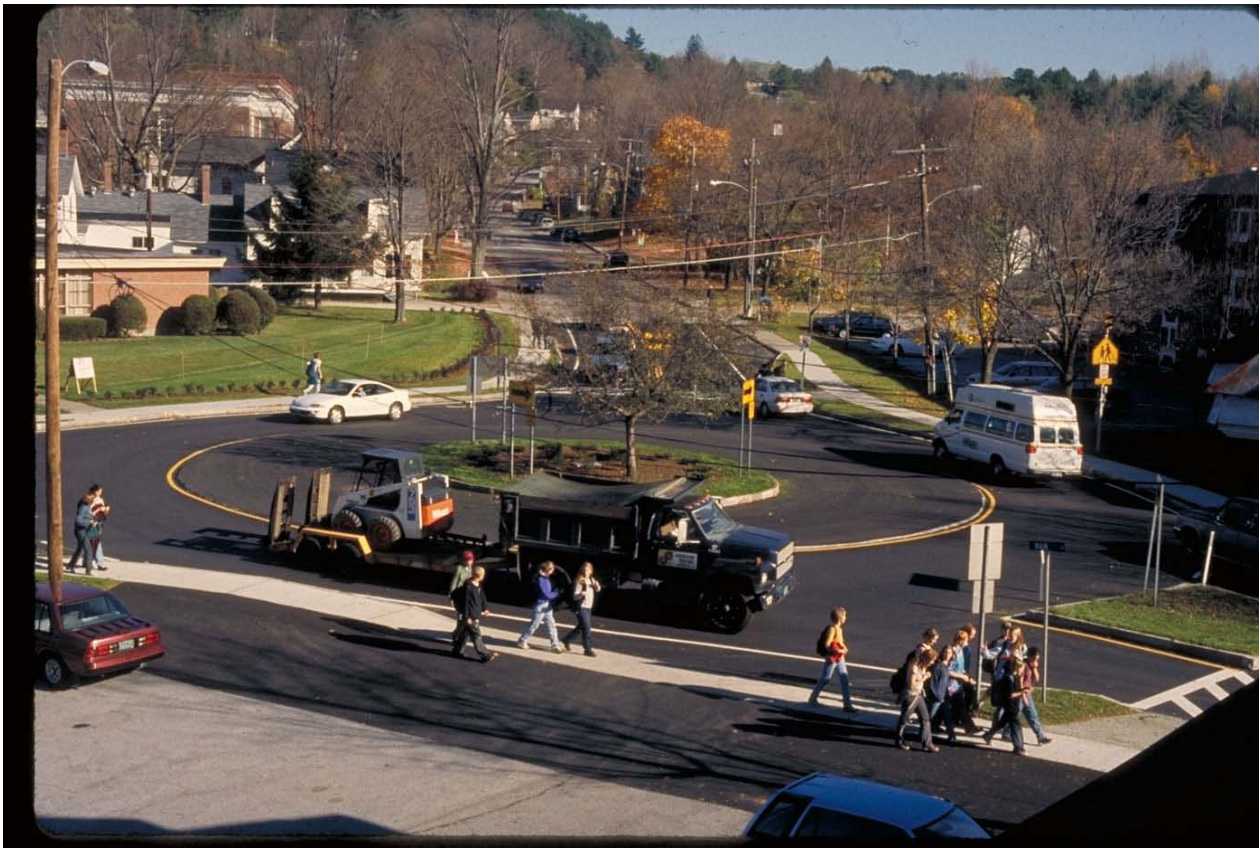
Another modern roundabout near a school in Montpelier, VT. Again, note that the entry widths are kept to no more than 13 feet, to ensure low speeds both at the pedestrian crosswalks and within the intersection. Photo: IMG0027.jpg
