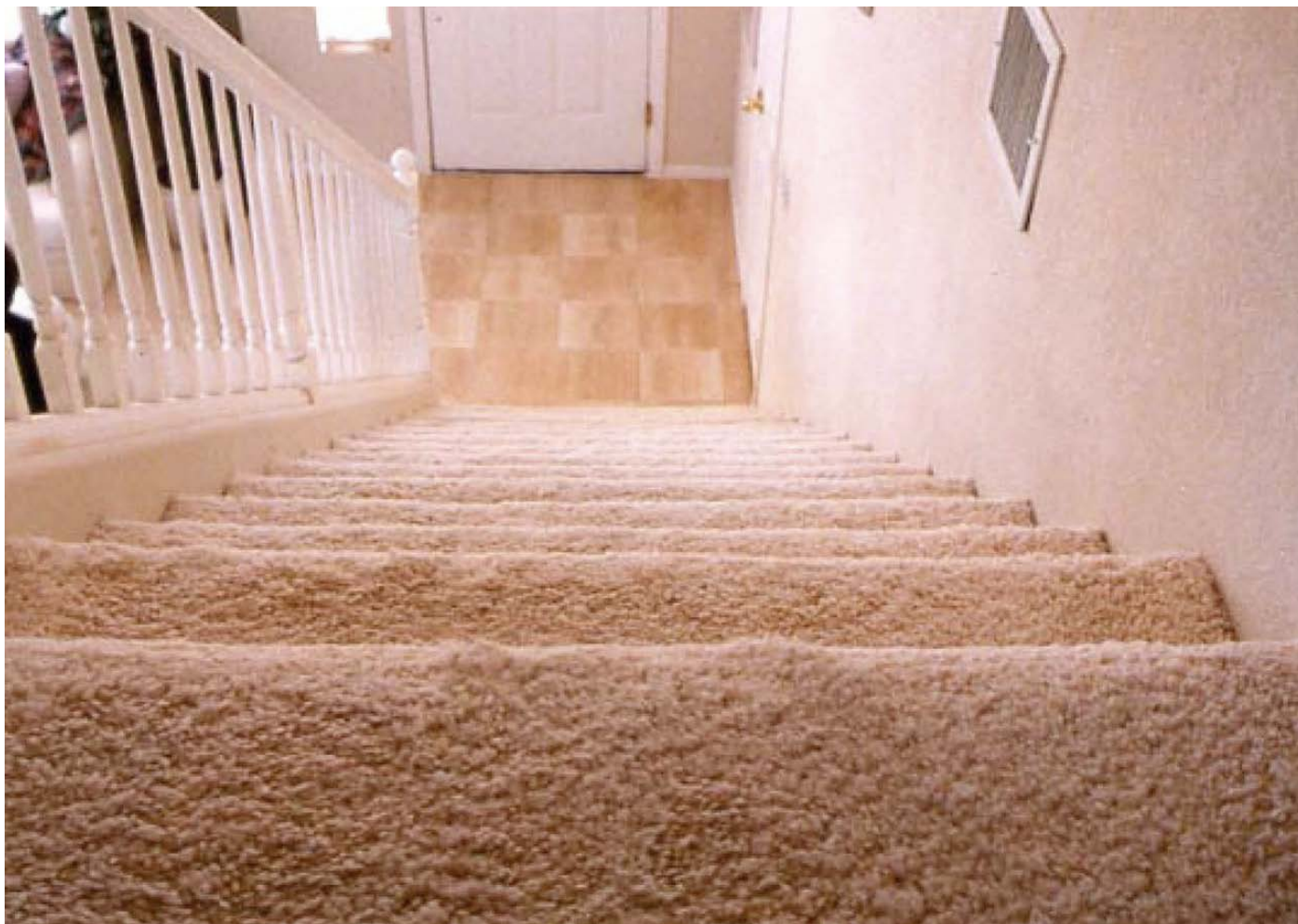
Figure 2. Typical Home Stair with Top-of-Flight, Tread Uniformity Defect
