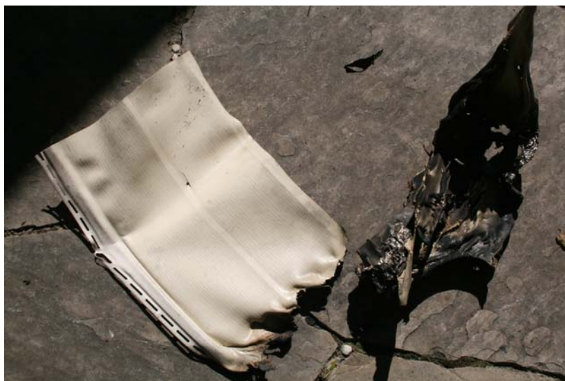
Figure 1 – Remains of vinyl siding fire
