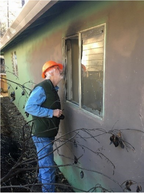
Complete failure of the glazing
