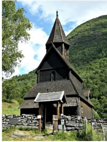
Heavy timber construction
