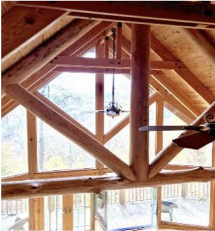
Log wall construction
