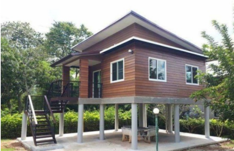
Figure 1. Usable unenclosed underfloor areas.
