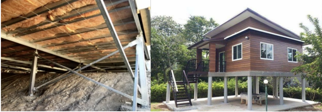
Figure 1. Noncombustible unenclosed underfloor areas.
