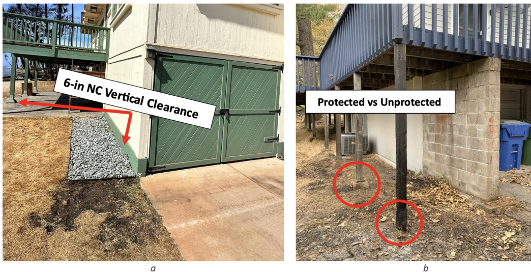
Figure 2. 6-in Noncombustible vertical clearance at the base of exterior walls and underfloor area columns: a. Lahaina Fire 2023 (Photo curtesy Milad Shabanian, IBHS), b. Glass Fire 2020 (Photo curtesy Steve Hawks, IBHS).
