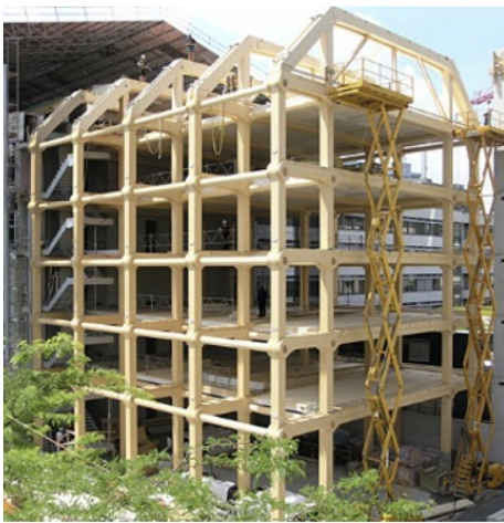
Post and Beam construction
