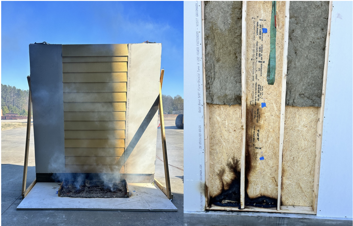
Figure 4. b. Typical exterior wall assemblies constructed on the exterior with noncombustible fiber cement siding material. Photo courtesy by Milad Shabanian, IBHS.
