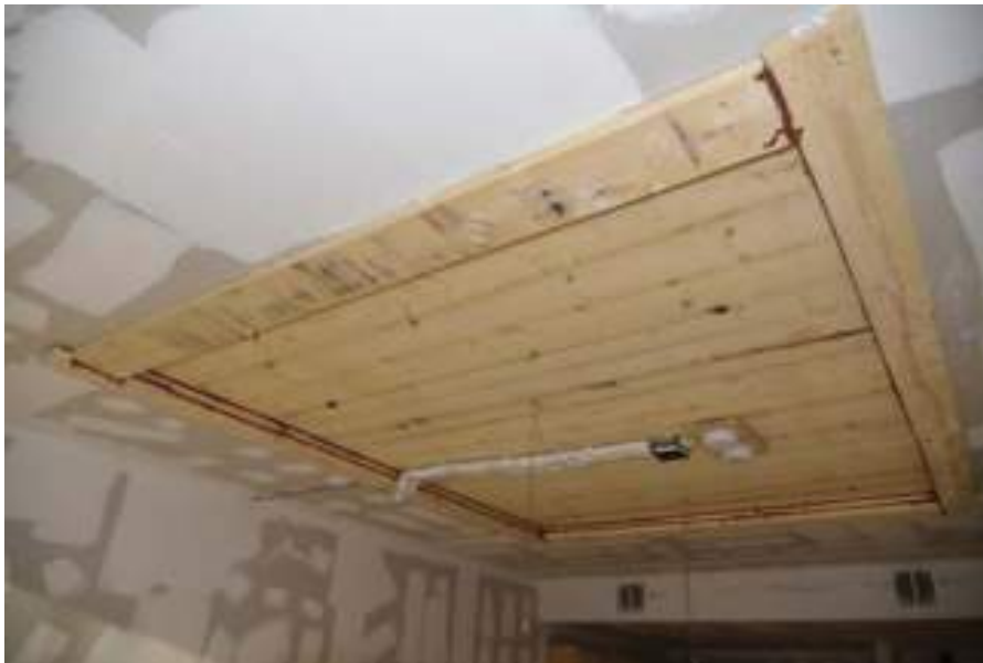
Figure 1: Exposed Ceiling for Test 2
