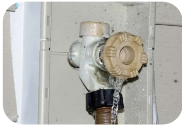
Leaks/Other Water Use
